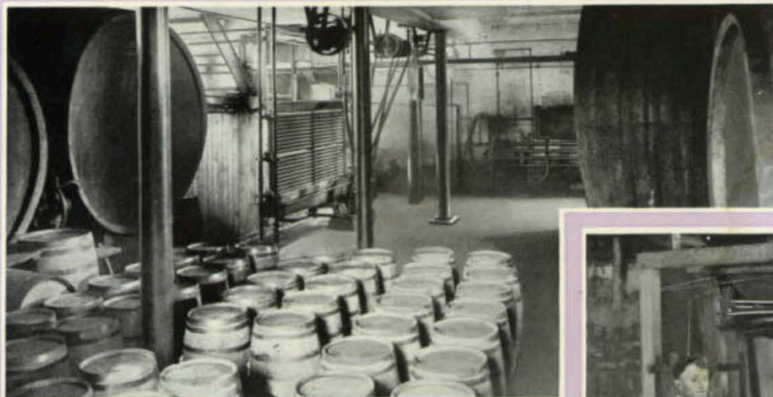
A CORNER OF THE VAULTS SHOWING JUICE-COOLING COILS IN THE BACKGROUND
